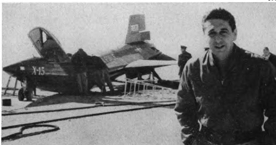
**TEST PILOT'S** big test came last November when fire broke out minutes after the X-15 was launched on its third power flight. Crossfield made landing uninjured but the impact fractured the ship's fuselage five feet behind cockpit.
